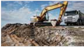
Truck / Heavy Equipment
